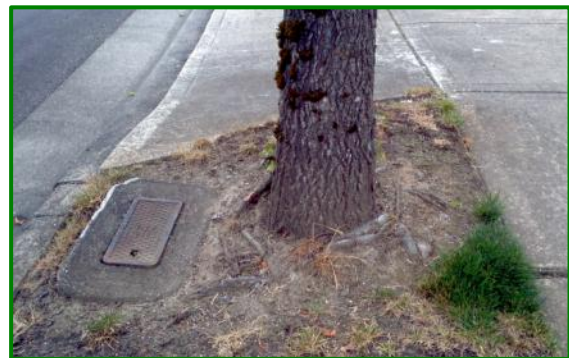
Tree is planted on water main line.
